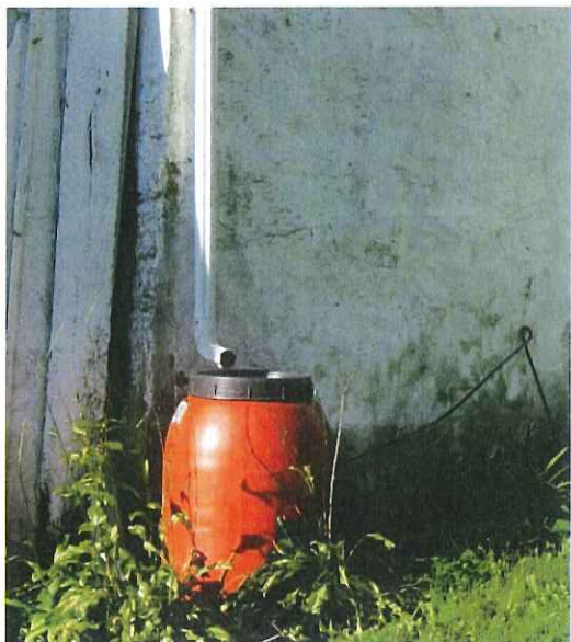
Rain barrels capture roof runoff. With a soaker hose attached, this BMP can also help your garden survive drier periods.
